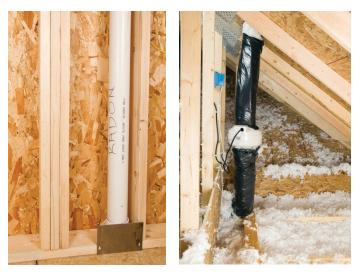
The best way to reduce the levels of radon in air is to install a radon mitigation system. A "certified mitigation specialist" should be called to install a system that fixes the problem. In most cases, this system involves drilling a hole in the basement floor and installing a vent pipe and a fan to reduce radon entry into the home.
