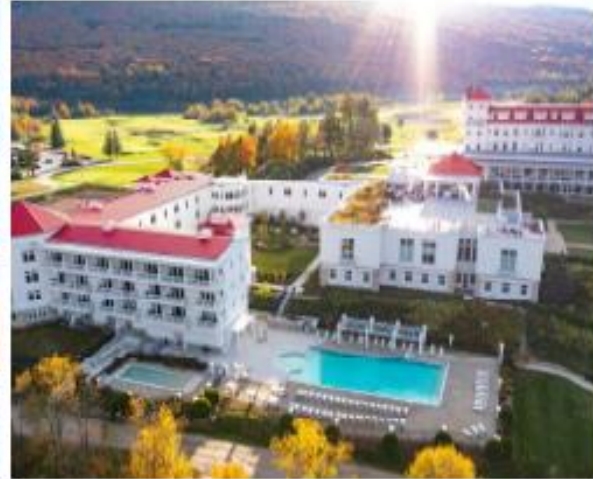
Omni Mount Washington Guestroom Addition Bretton Woods, NH
