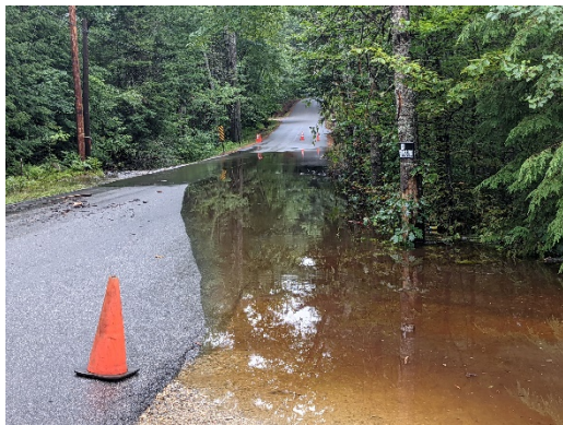
Photos of Richmond Road in Troy in July of 2021
